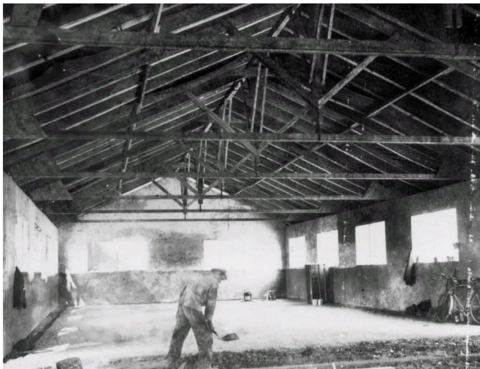
While the enlisted Mess Hall was being built...
