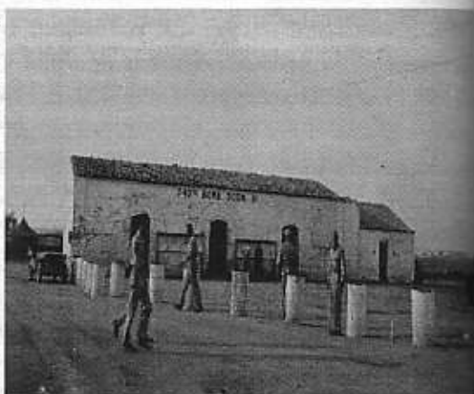
Operations Headquarters, Italy
